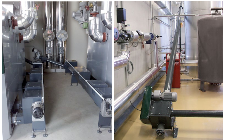
This image shows the ash containers of a 2 HERZ boiler cascade solution connected via the screw system.
