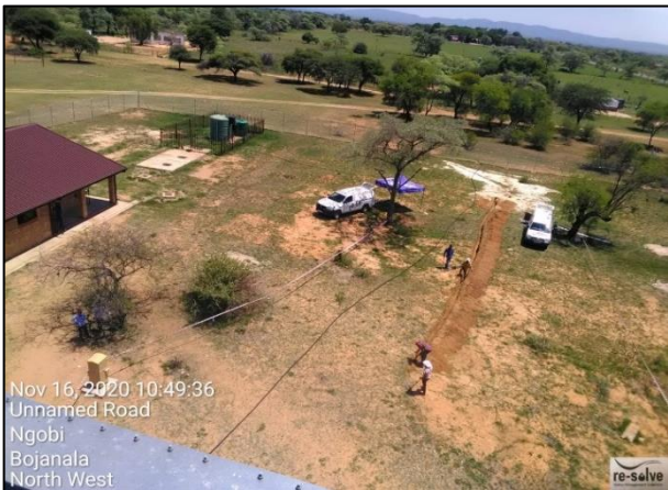
Installation of the 50mm HDPE pipe and electrical cables
