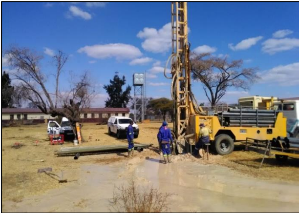
Drilling of new borehole at Ngobi Primary School
