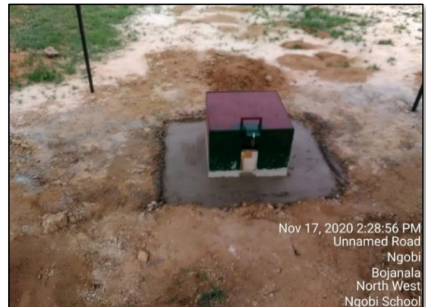
Borehole pump case post installation
