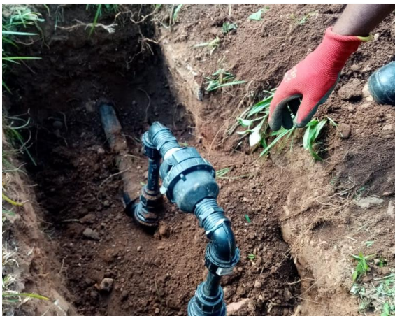
Newly installed 20mm sub-meter
