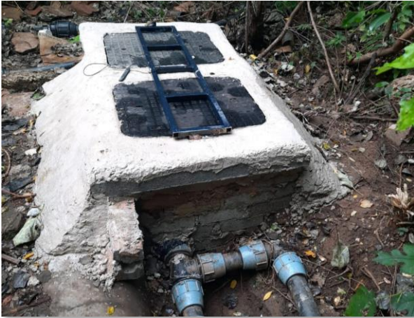
Newly built PRV chamber
