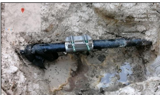
Leak Detection Repairs
