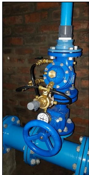
Interior and Exterior View of Constructed PRV Chamber
